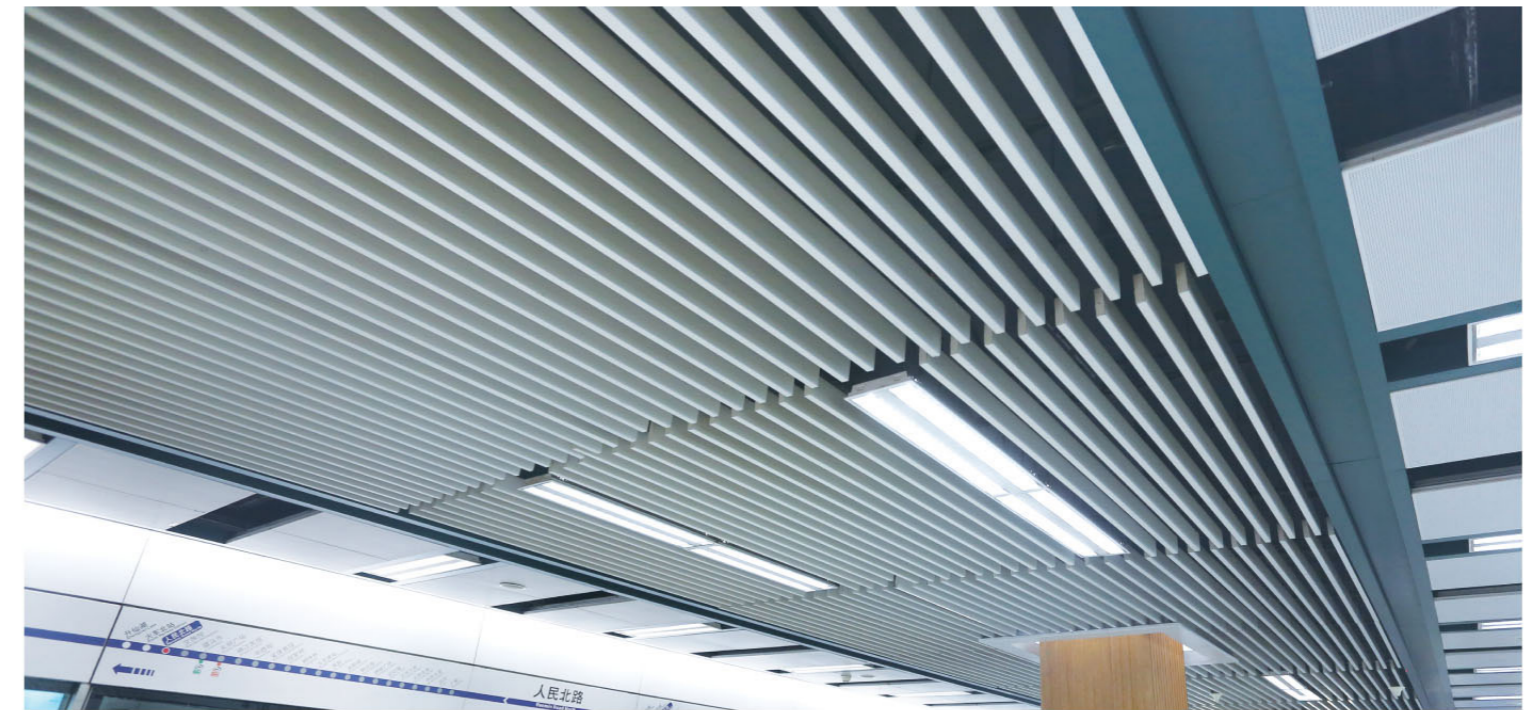
型材方通安装实例 Profiles Square Tube Installation Sample
